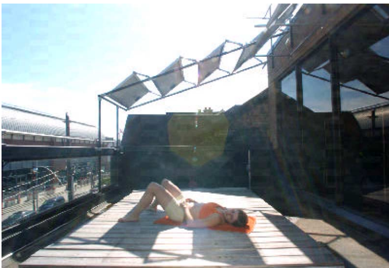
Fig. 2. After capturing the sunlight's energy, the light is split and diffused, creating a pleasant mix of sun and shade for the occupant.
