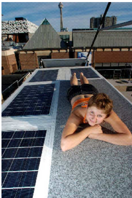
Fig. 4. Agata Jaworski, a designer of the ETRC, enjoys the Flexible Solar Membrane on the roof of the mechanical room.
