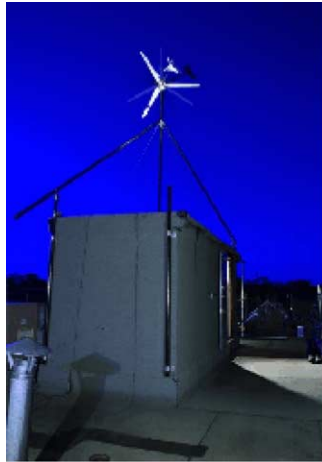
Fig. 5. The Urbine: Canada's first rooftop mounted urban wind turbine. The frame of the urbine also supported the outdoor shower, cooling occupants as they relax on the Flexible Solar Membrane.
