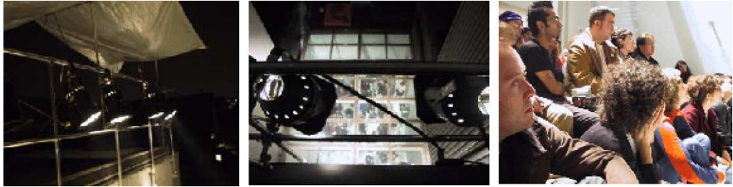
Fig. 6. The Natural Artificial Lighting System of the ETRC includes large ceiling windows to let light in and white opaque walls that trap the light once inside. This system transforms a dark, rainy evening into one which appears bright and filled with daylight.
