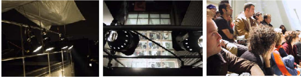
Fig. 6. The Natural Artificial Lighting System of the ETRC includes large ceiling windows to let light in and white opaque walls that trap the light once inside. This system transforms a dark, rainy evening into one which appears bright and filled with daylight.
