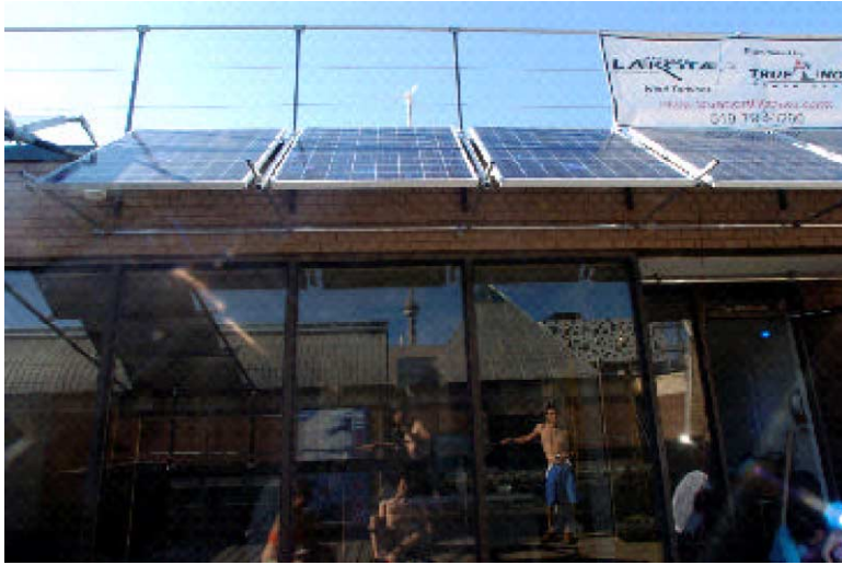
Fig. 1. The Solar Awning not only captures the sun's energy, but provides a shaded outdoor area for the occupants of the building.
