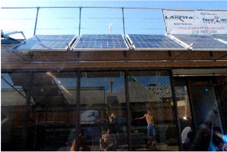
153 Fig. 1. The Solar Awning not only captures the sun's energy, but provides a shaded outdoor area for the occupants 154 of the building.
